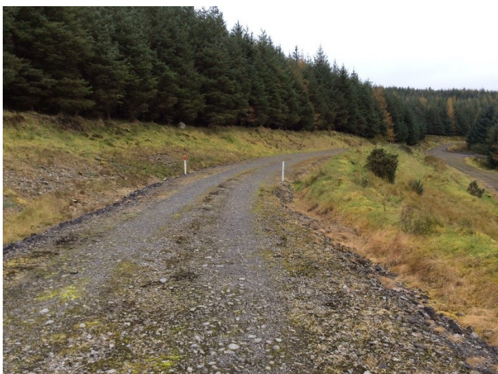
Plate 24: Hardstand for T8, looking SE.
