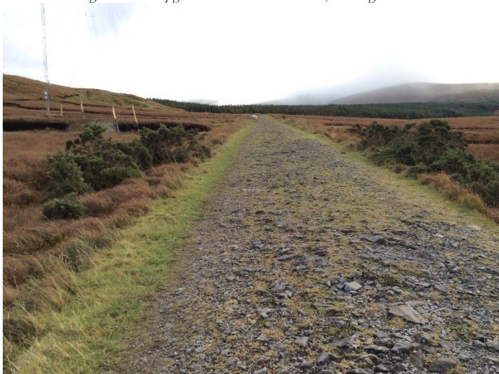
Plate 8: Existing Road for upgrade looking E towards T5.
