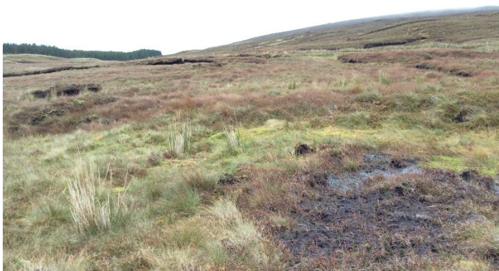
Plate 30: Hardstand for T12, looking NE.
