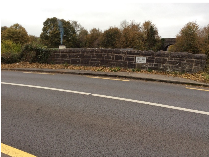
Plate 48: Railway bridge CH29 on Proposed Grid Connection Route north of Collooney.
