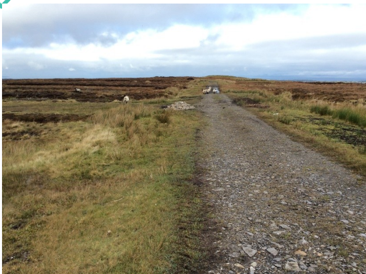
Plate 16: Existing Road for upgrade south of T2, looking NW.
