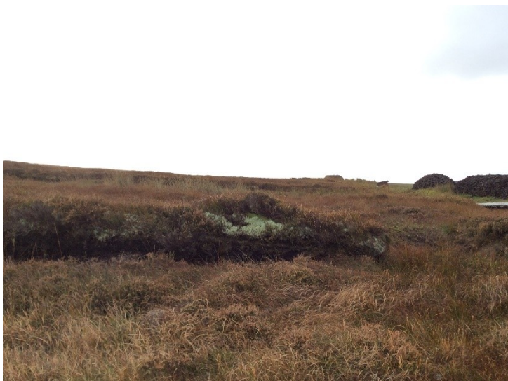
Plate 2: T1 hardstand, looking SE.
