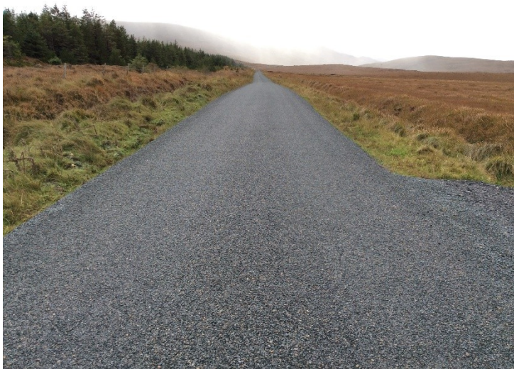
Plate 11: Public road for upgrade to E of T1, T3 and T5, looking SE.
