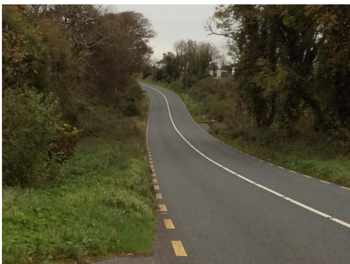
Plate 45: West end of Proposed Grid Connection Route on public road, looking E.
