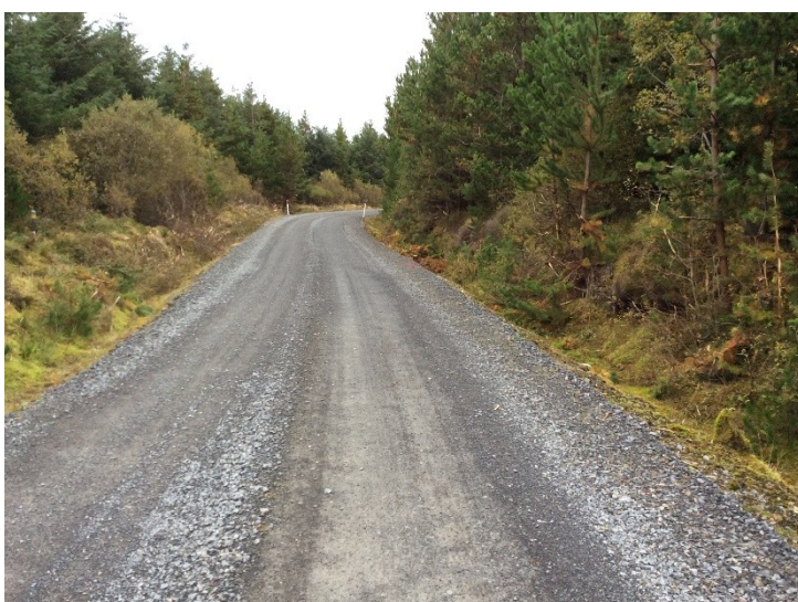
Plate 27: Existing Road to west of T10, looking NE.
