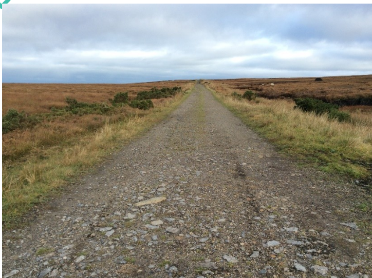
Plate 7: Existing Road for upgrade south of T1 and T3, looking NW.
